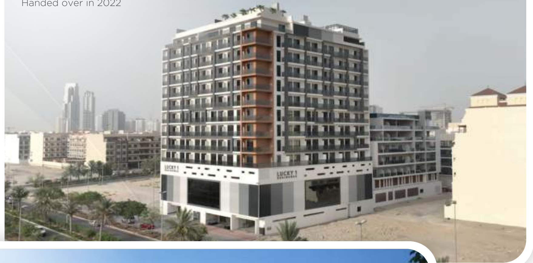
Lucky Residence Handed over in 2022
